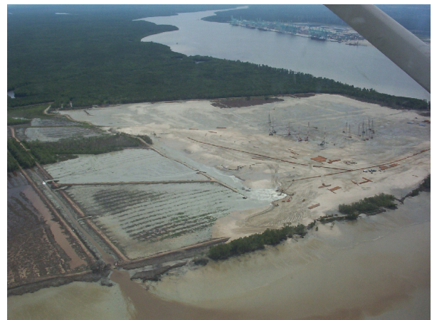
Tanjung Bin reclamation site
