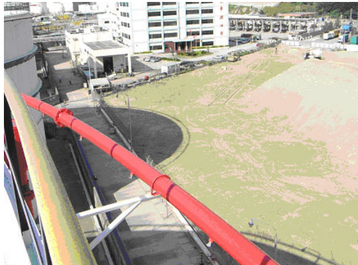
View northwards from Oil Tank
