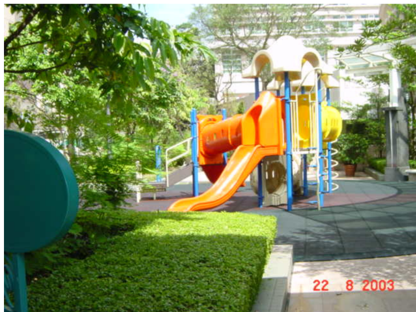
Completed Playground near to repaired slope
