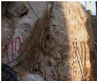
Removal of unstable boulders
