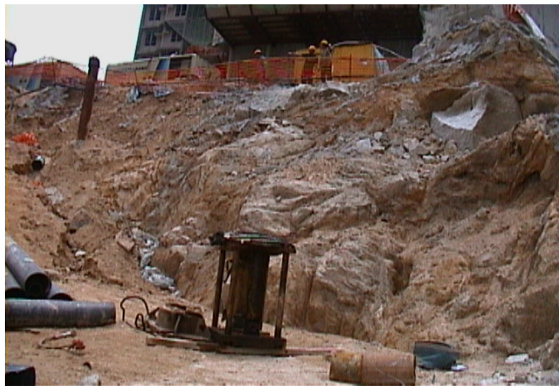
Rock excavation for proposed site formation
