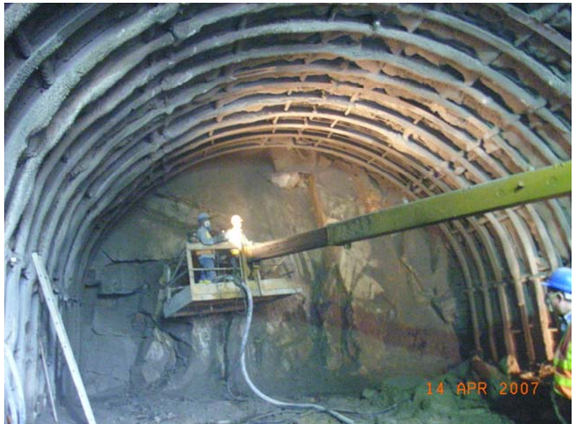
Adit tunnel excavation underway showing temporary support system
