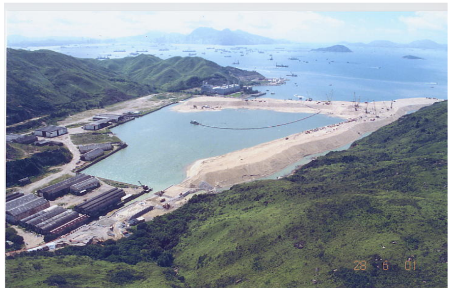
Aerial view of Penny's Bay during construction - looking east
