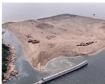
Close-up of western seawall
